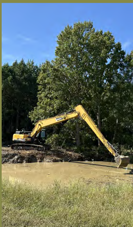
An excavator removes sediment that has washed into an irrigation pond over the years, increasing the storage capacity.
