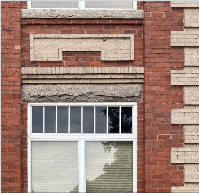
The characteristics of the blonde and red brick of the Wakelon School contrast the stone lintels and sills. Maintaining and preserving characteristics like this are appropriate. Photograph by Loggia Preservation, 2025.
