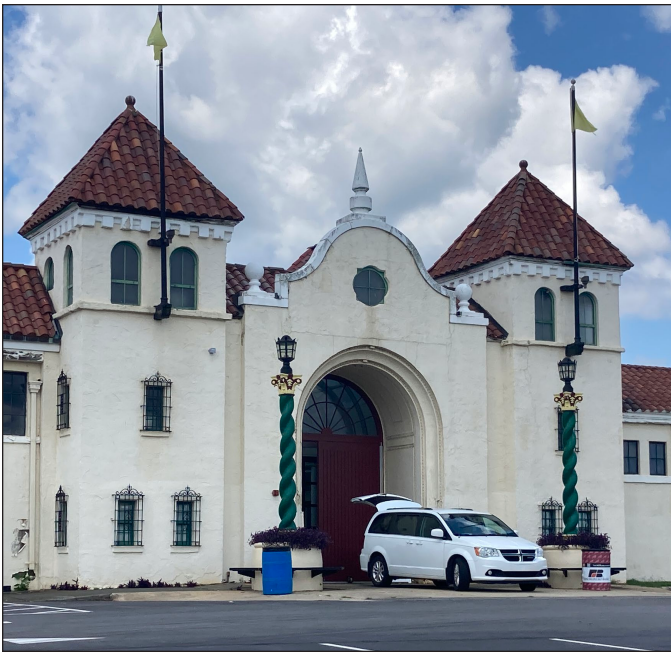
The North Carolina State Commercial and Agricultural Building has a myriad of masonry features like exterior stucco, a red clay tile roof, a masonry parapet, and other decorative masonry elements. Photograph by Loggia Preservation, 2025.
