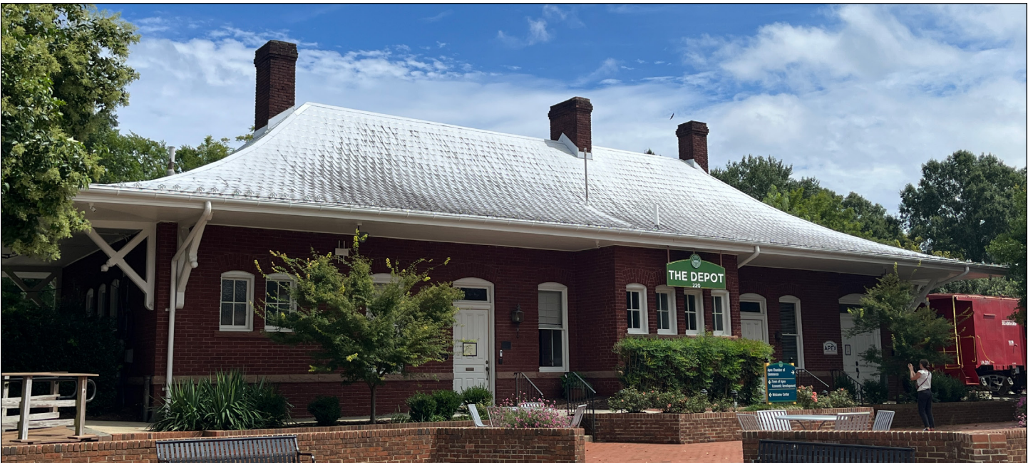
The Apex Union Depot features a distinctive bell-cast hipped roof clad in individually pressed metal shingles. Photograph by Loggia Preservation, 2025.
