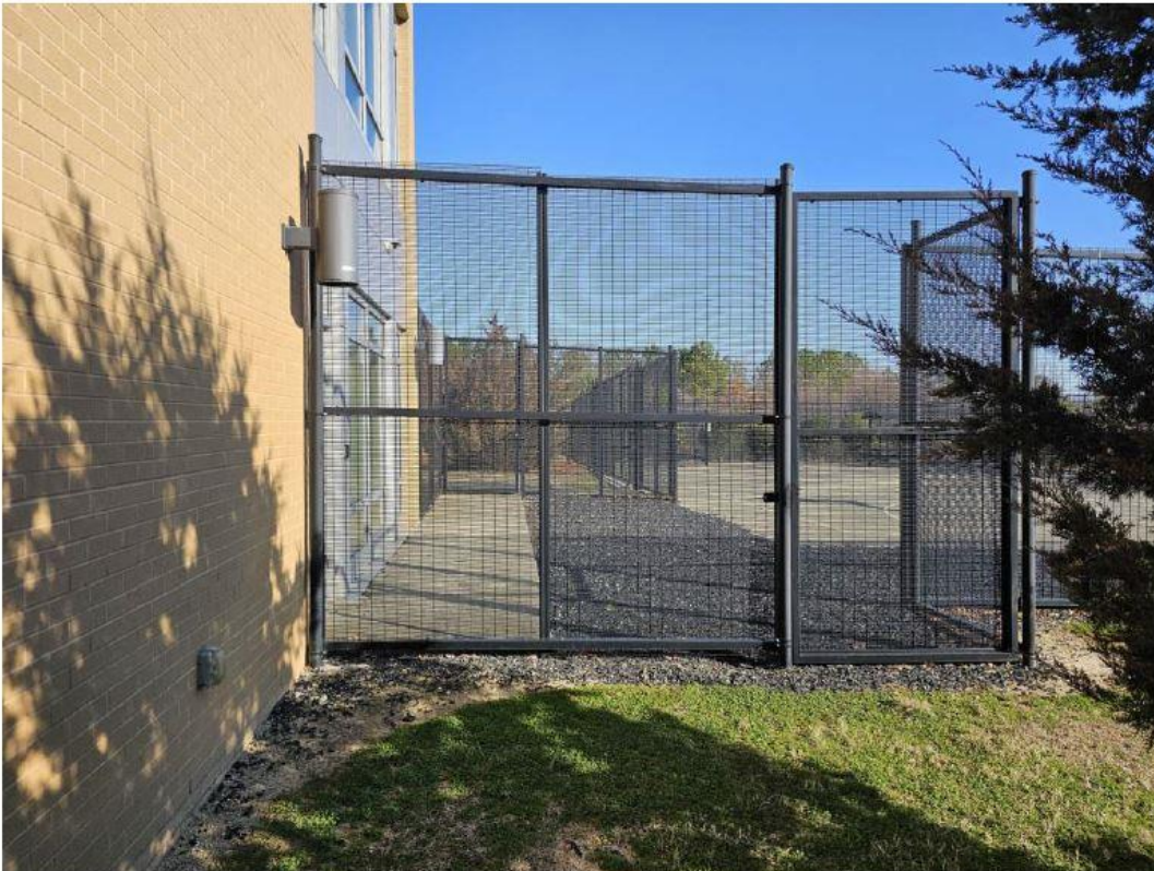
EXISTING SWING GATE
