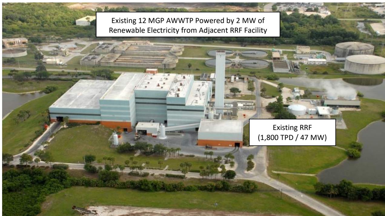
Figure 1. Hillsborough County, Florida RRF Facility provides 2 MW of Renewable Electricity to 12 MGD AWWTP and other adjacent Public Works
