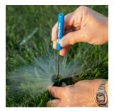
Sprinkler head adjustment for less water waste.
