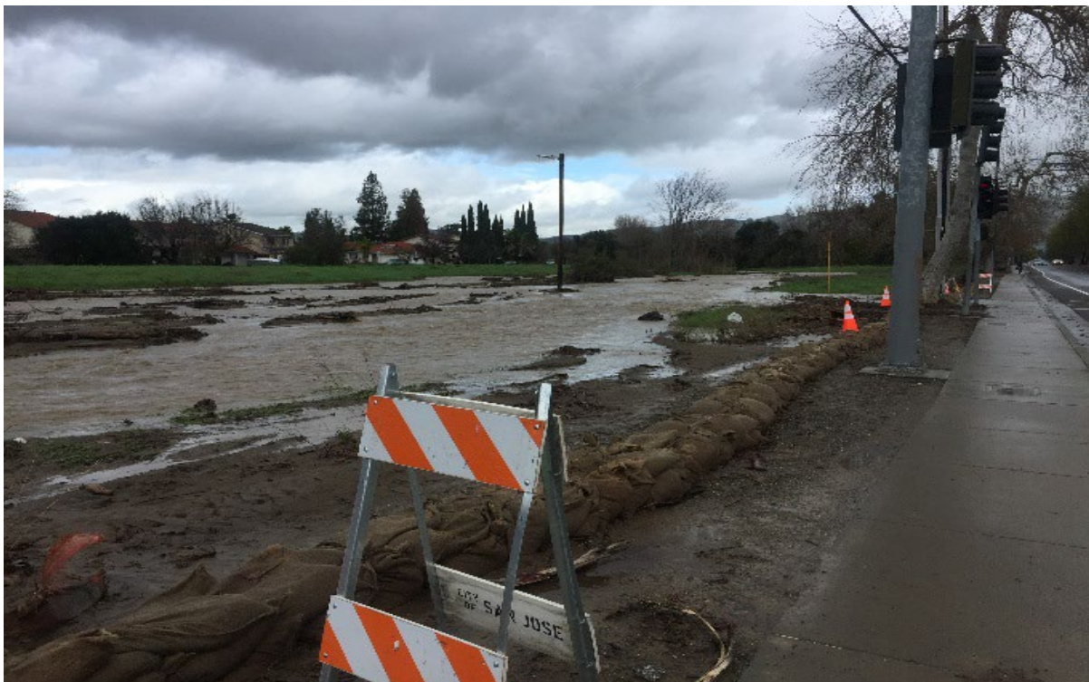
Figure 3-5: Mabury Bypass January 2017 – sandbags to prevent flooding of Mabury Rd
