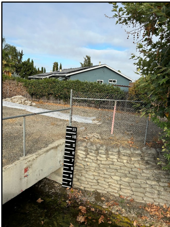
Reach 12 – Upstream Cropley Road entrance to the 400-foot culvert with visual gauge and web cam
