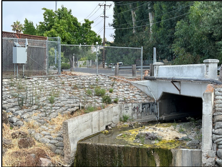
Reach 12 – Looking upstream at the Old Piedmont Road culvert and drop/grade control structure with ALERT stream gauge
