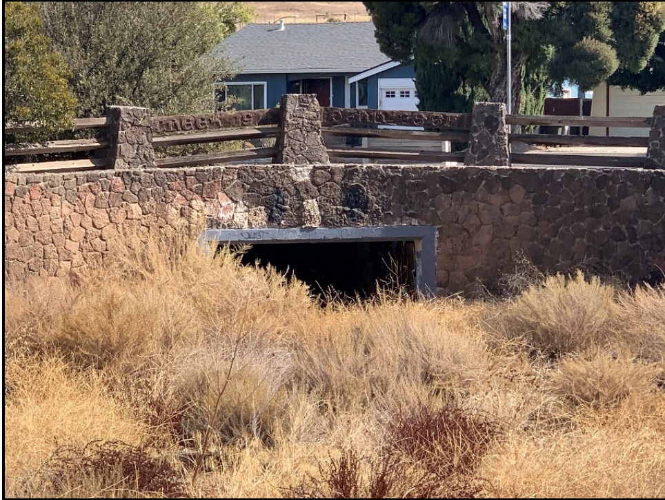
Reach 12 – Looking from downstream of Piedmont Road at exit of approximately 400-foot culvert that crosses under Cropley Road and Piedmont Road.
