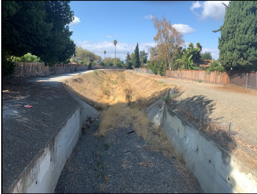
Reach 9 – Looking downstream from Morrill Avenue at concrete transition to excavated earth channel
