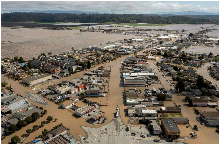
March 2023 flooding along Pajaro River
