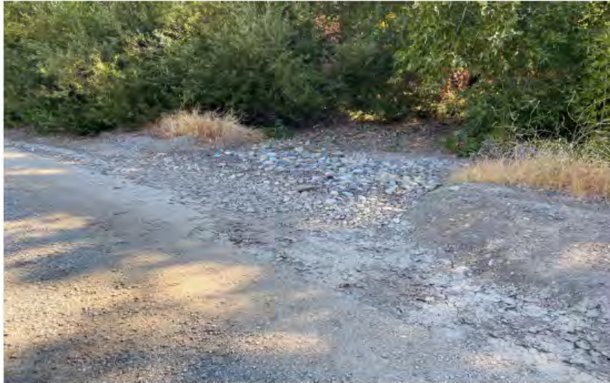
PICTURE 1: Inspection Date: 07-27-2021 - Looking: UNKNOWN
