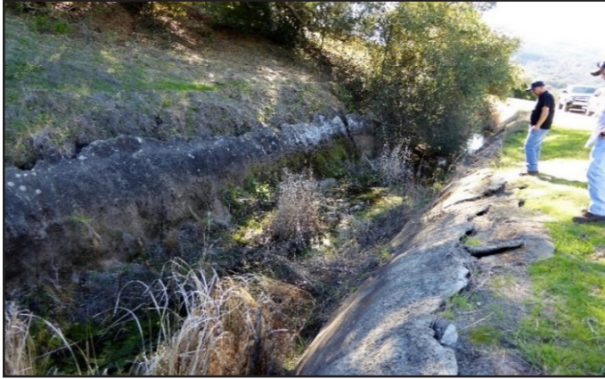
Cracks and separated lining in the canal
