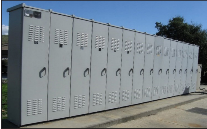
Motor control center switchboard
