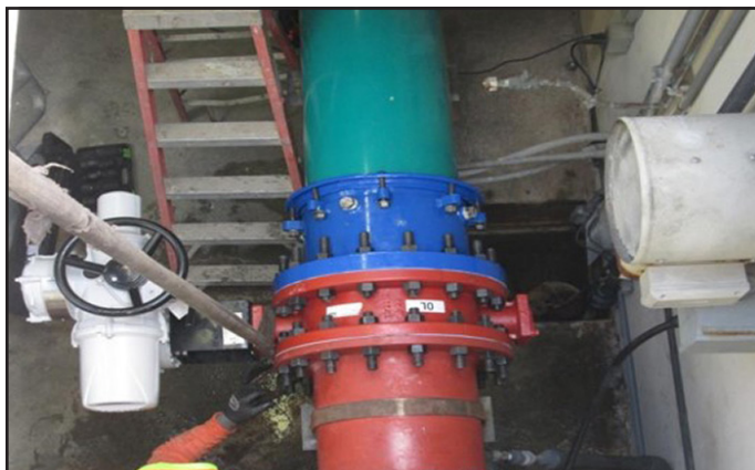
A typical rehabilitated line valve assembly
