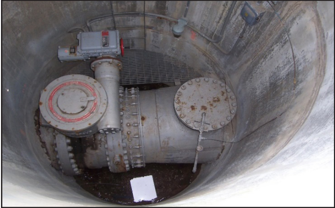
Typical steel pipeline in line valve vault
