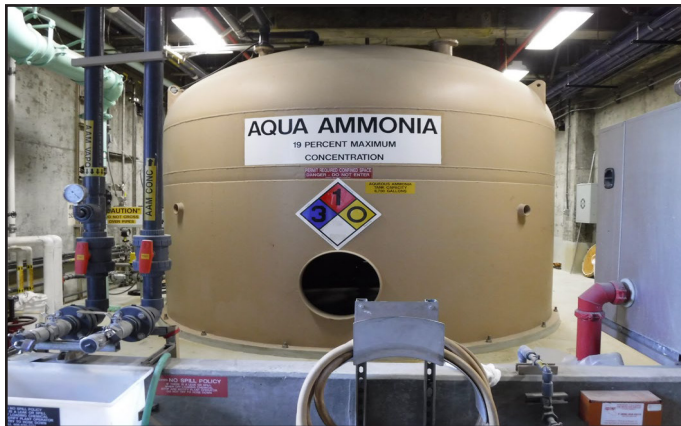
Rinconada Water Treatment Plant Aqua Ammonia Tank
