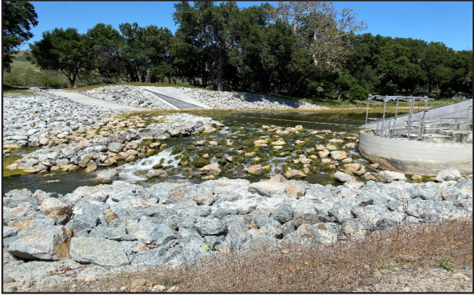
Upstream view of Coyote Percolation Dam, fish ladder, and rock slope protection
