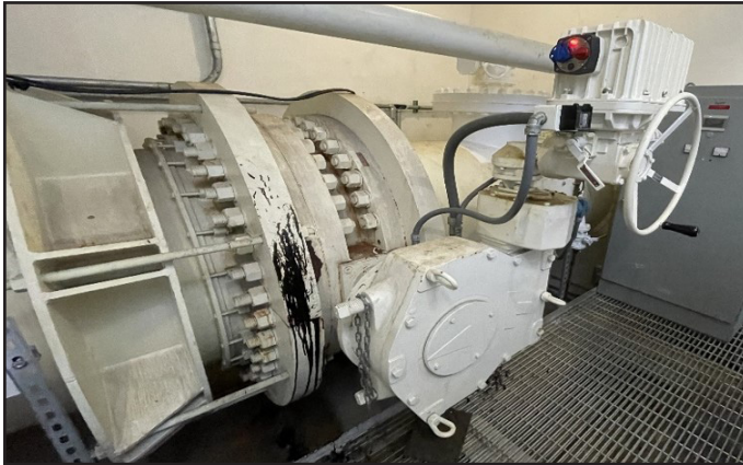
A valve that to be replaced as a part of the project
