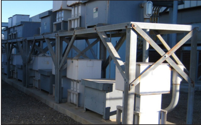
ASD motors at the Coyote Pumping Plant
