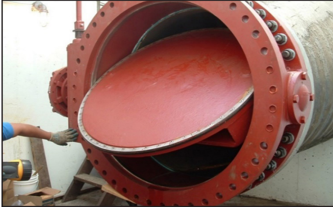
Valve installation in the Piedmont Line Valve Vault; Similar projects will be carried out at treated water transmission facilities according to the asset management plan
