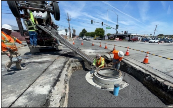
12" RCW turnout connection at the intersection of Monterey Road and Luchessa Ave. in Gilroy, CA
