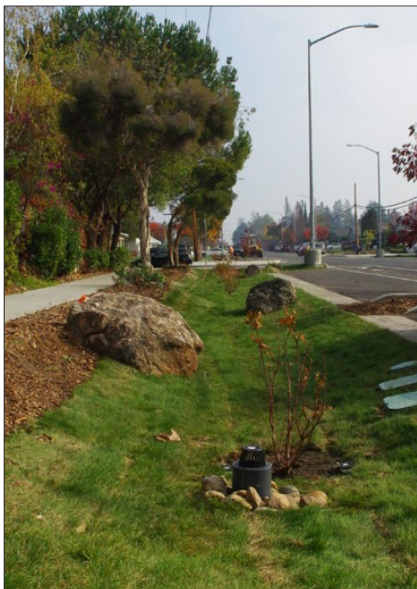
Bioretention Basin. Photo: Valley Water
