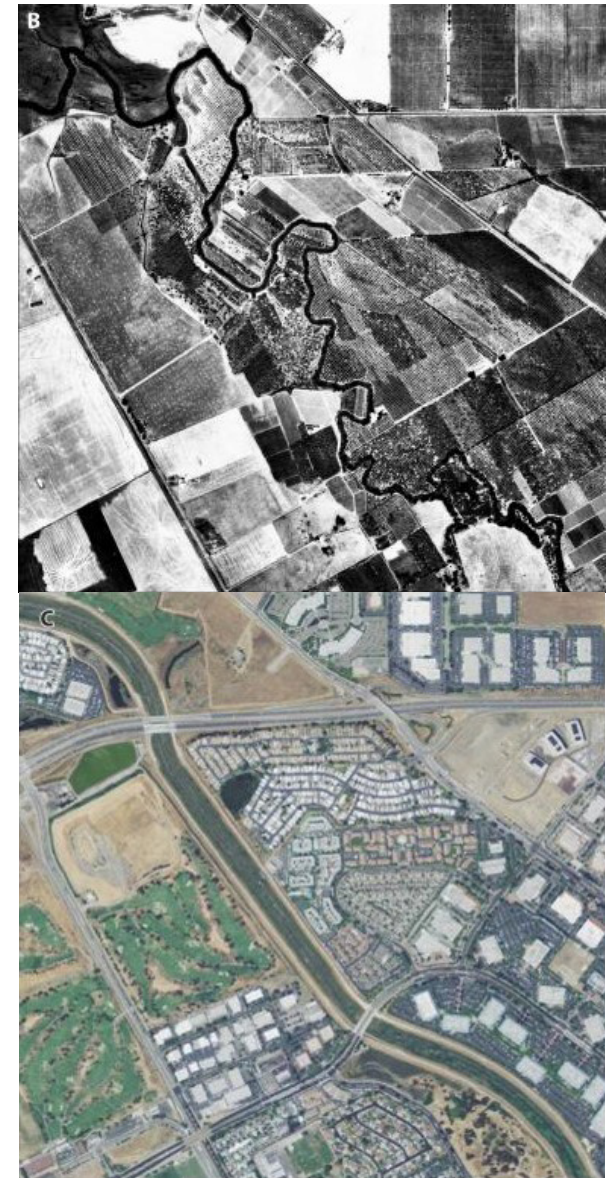
Figure 2-2: Comparison of historical (top) and contemporary (bottom) lower Guadalupe River, illustrating its channelization and loss of adjacent riparian forest (Beller, Salomon, & Grossinger, 2010)
