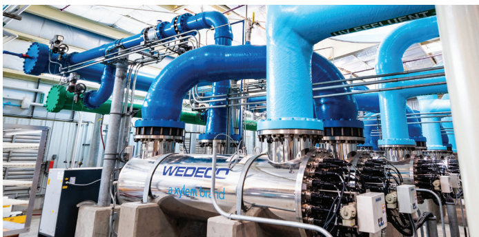
Silicon Valley Advanced Water Purification Center UV disinfection system.
