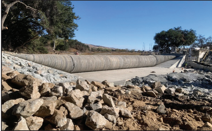
Phase 1 of the Coyote Percolation Dam has been completed, and the image shows the newly installed inflated bladder dam
