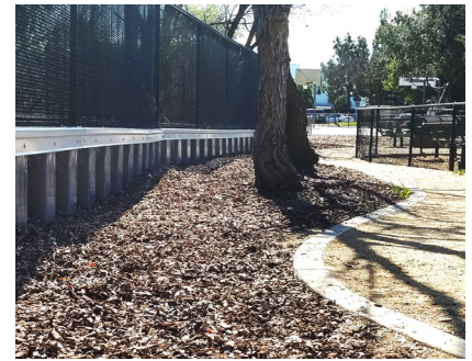
Vinyl sheet pile wall installed next to Rocksprings Park. Under the preferred alternatives for Reach 8, the sheet pile will be extended and raised.
