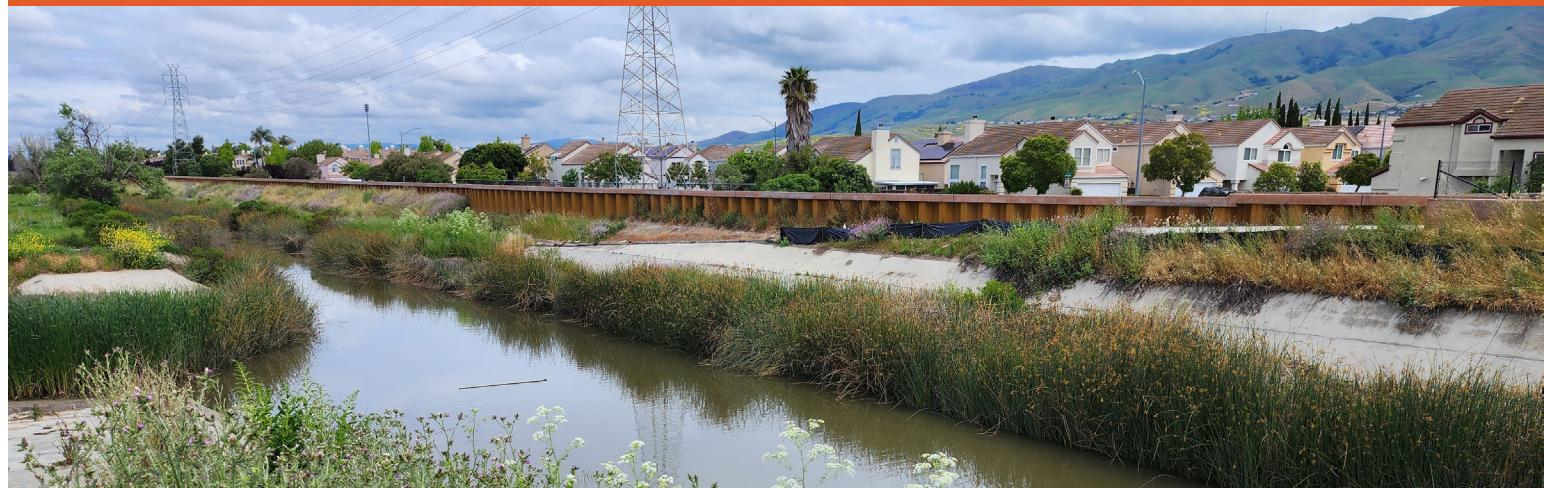
In summer 2023, Valley Water completed the Lower Penitencia Creek Improvements Project, which provides continued flood protection for residents and businesses along a one-mile stretch. Valley Water installed about 7,200 feet of interlocking sheets of steel and a new levee to create 1.3-miles of flood protection along the creek.
