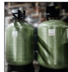
FRIT San Jose Town and Country Village LLC: Cooling Tower Makeup Water Softener System.
