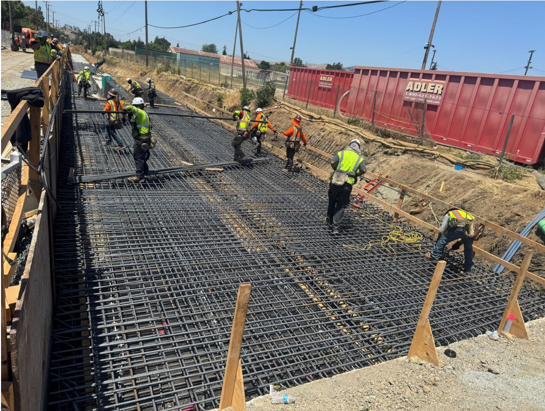
Installation of reinforced concrete box culvert at Hale Ave.
