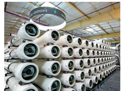
Water Purification Center reverse osmosis.
