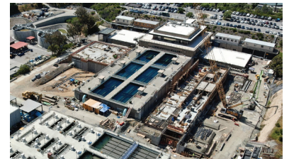
Phase 4 construction progress includes building structures that will make up the Dual Media Filters, Chlorine Contact Basin, Ozone Generation Building, and Liquid Oxygen Facility.
