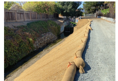
Streambed and banks stabilized on Regnart Creek as part of the Stream Maintenance Program.
