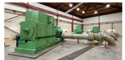
Existing pump gallery at the Coyote Pumping Plant. The existing pump motor on the left side of the picture will be rehabilitated as a part of the Coyote Pumping Plant Adjustable Speed Drive Replacement Project.
