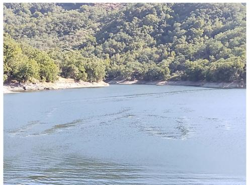
Figure 4: Almaden Reservoir bubble pattern following diffuser maintenance.
