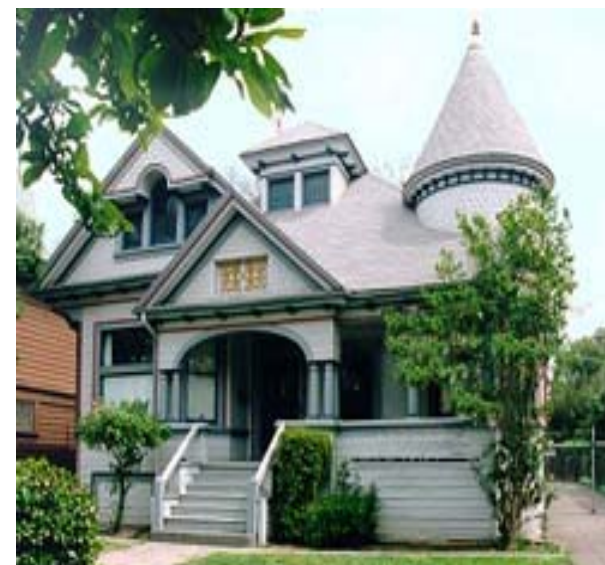
(#2) 1330 North Hunter Street—Queen Anne house, constructed in 1899.
