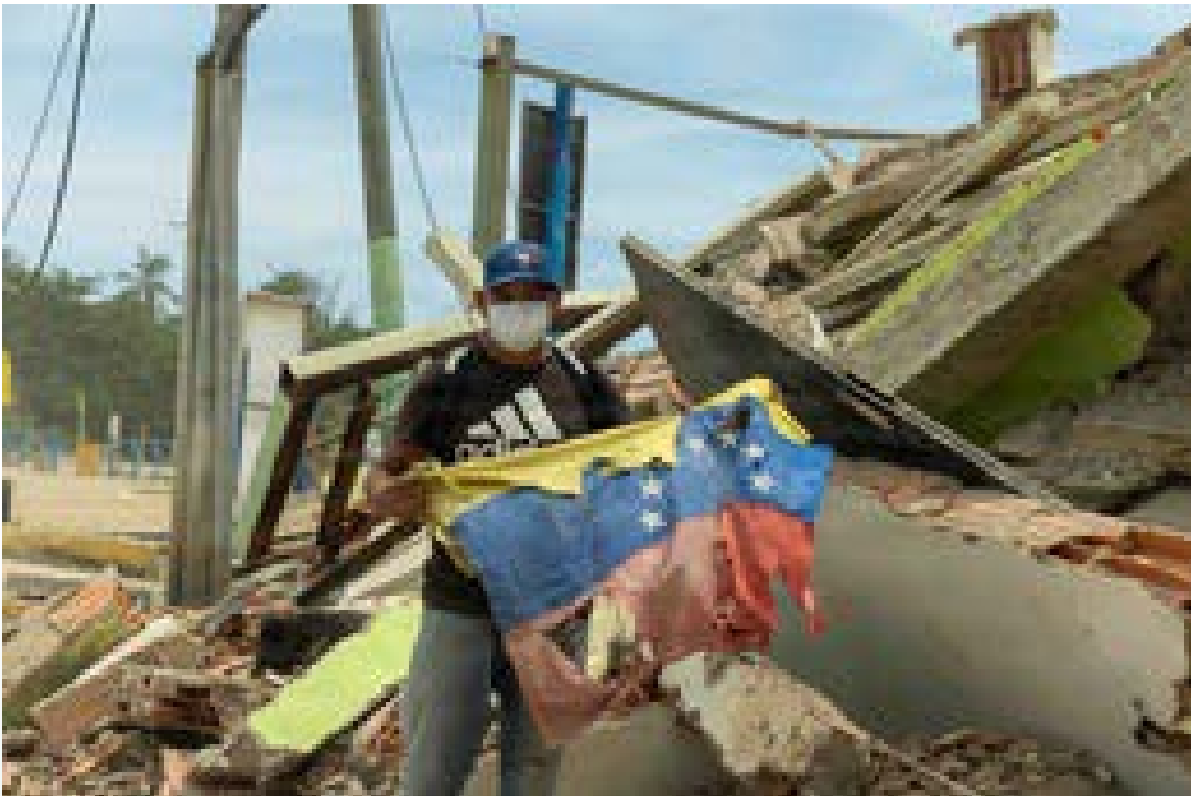
—Photo By Lance Cpl. Allison White | A Venezuelan citizen holds a national flag next to his damaged restaurant following an earthquake in La Guaira, Venezuela June 28, 2026. At the direction of U.S. Southern Command, assigned to U.S. Military forces are supporting Department of State-led U.S. disaster assistance to the people of Venezuela in the aftermath of June 24, 2026, earthquakes, (U.S. Marine Corps photo)
