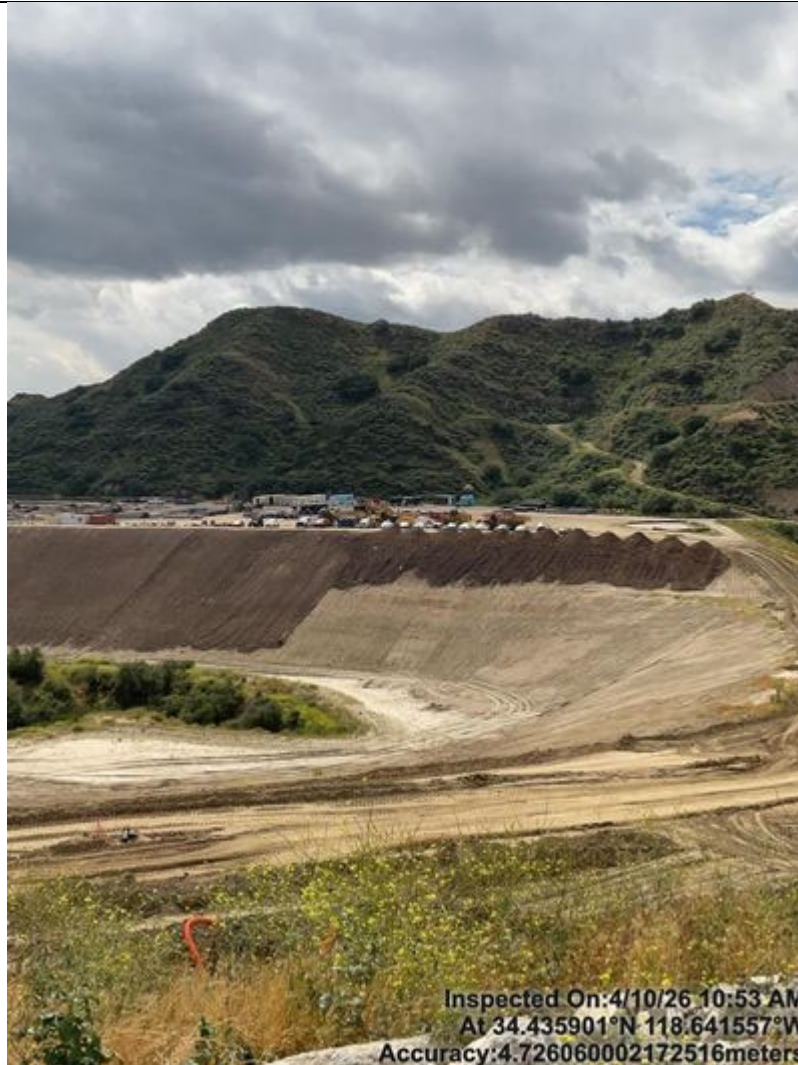
Photo 86 Slope being track walked with fresh media at the northeast end of the Site
