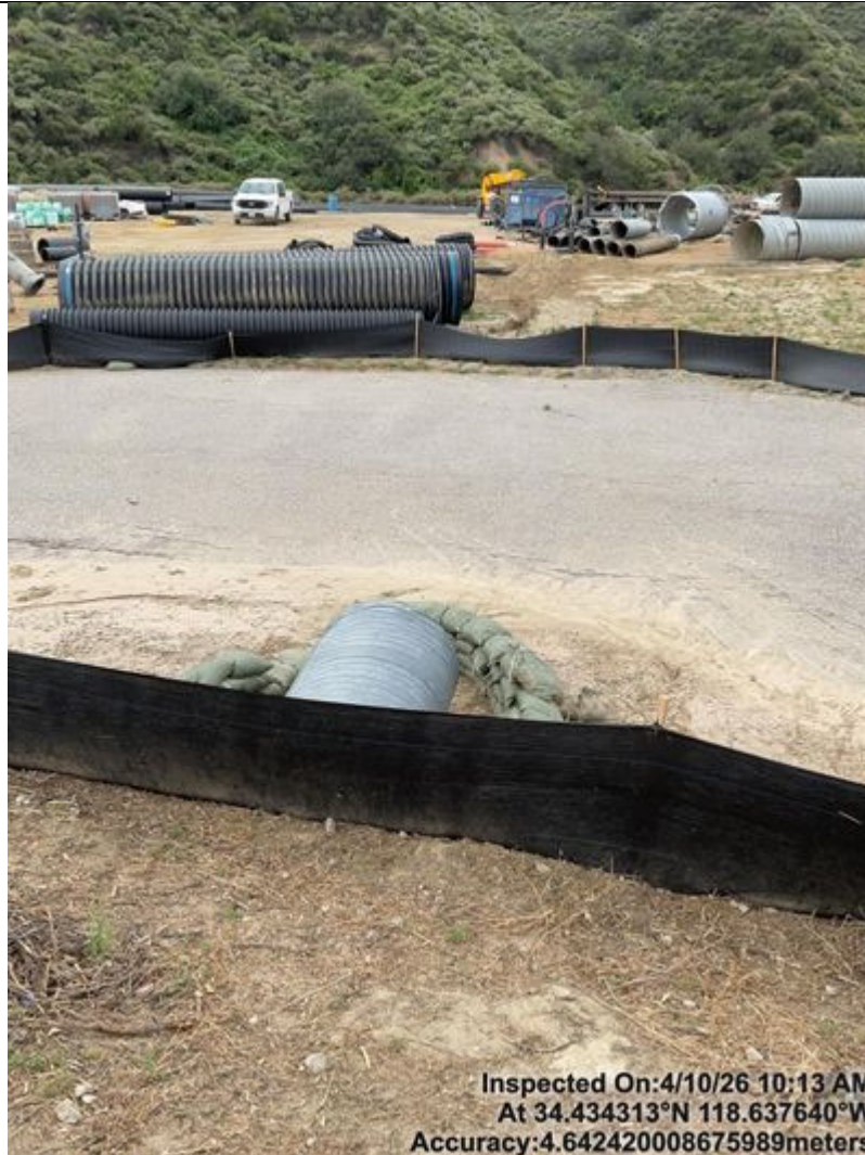
Photo 27 Culvert with sandbags at the equipment storage area/pipe lay down yard
