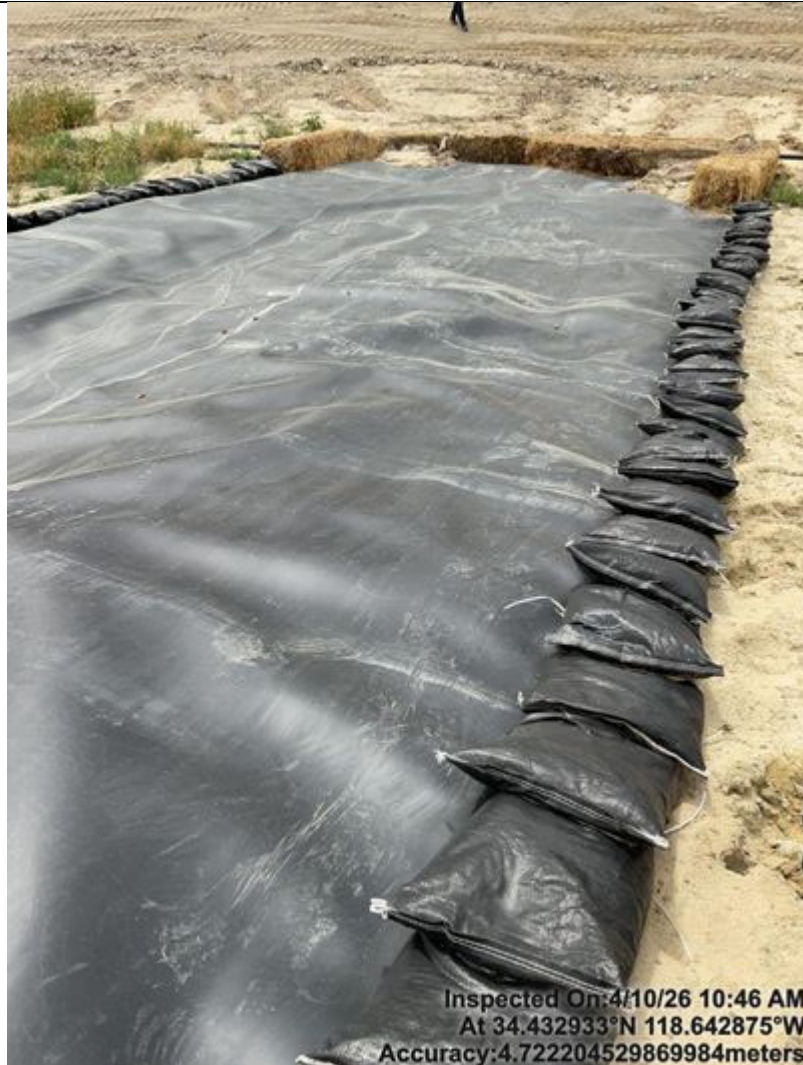
Photo 78 Close up of erosion control BMP
