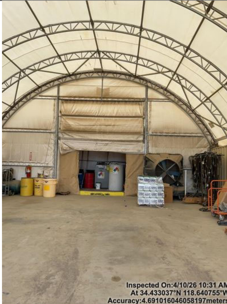
Photo 59 Inside the covered maintenance area
