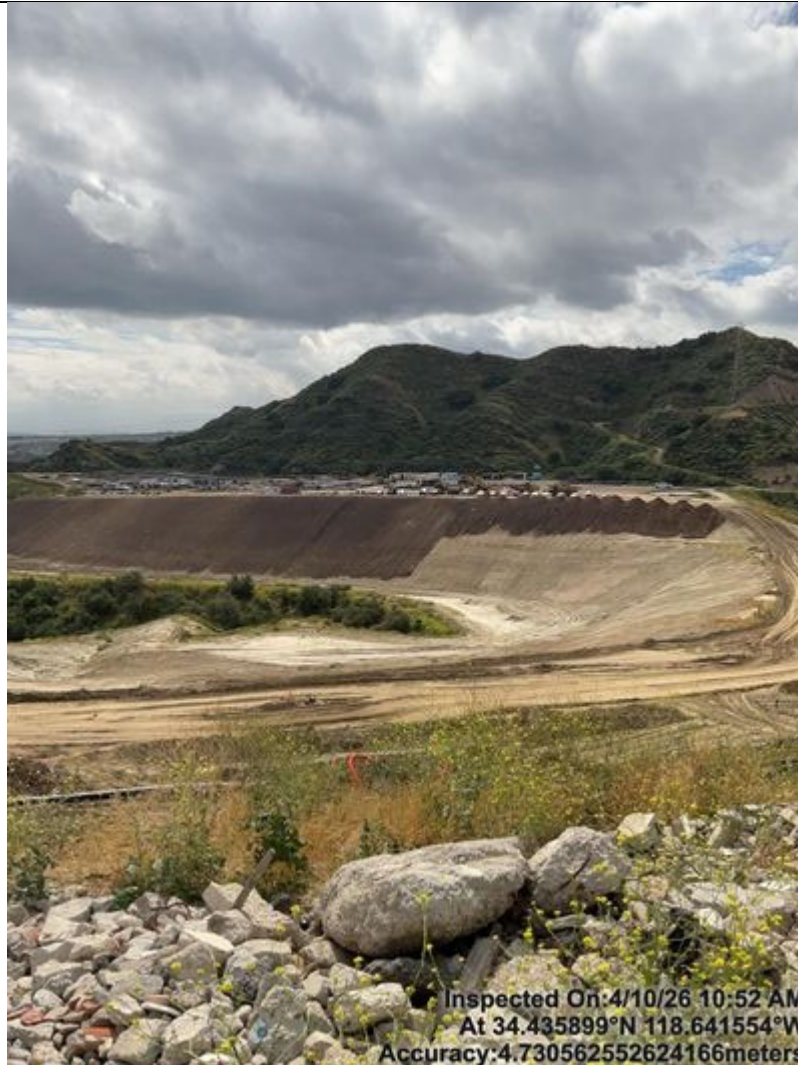
Photo 85 Slope being track walked with fresh media at the northeast end of the Site
