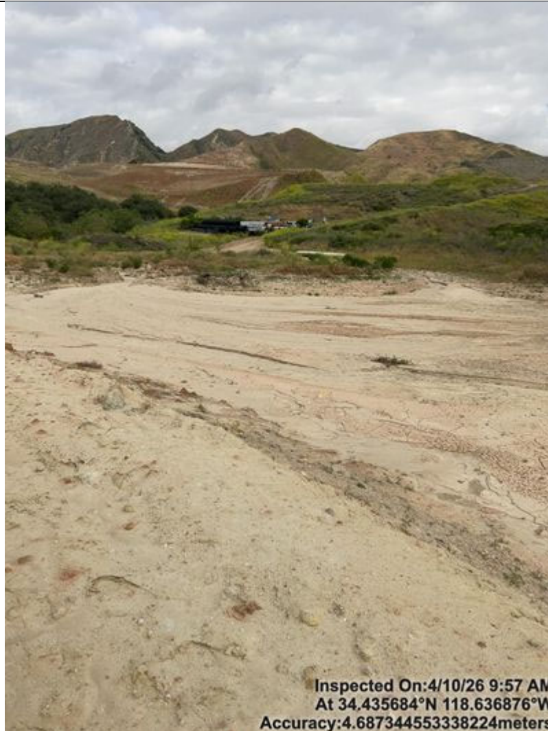
Photo 12 Sub basin 3 installed upgradient of the East Basin
