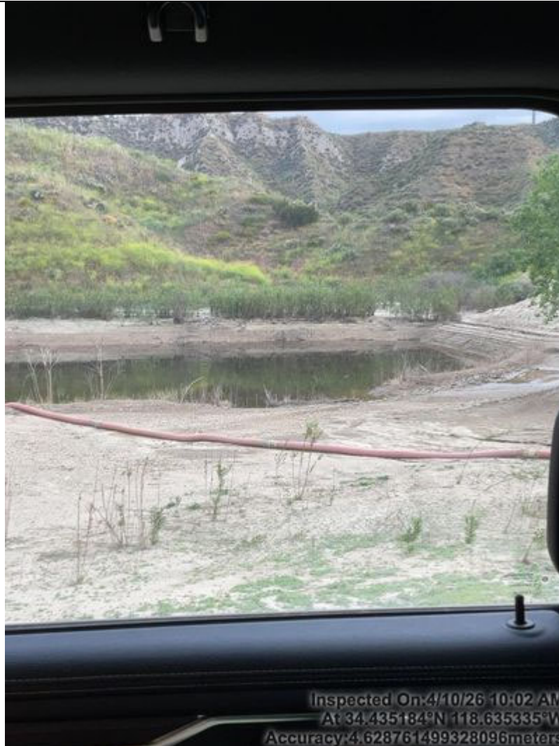
Photo 15 A view of the water in sub basin 2 of the East Basin
