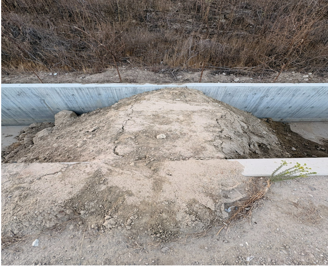
Photo 9. Check Dam in Box Culvert Near West Toe of Landfill
