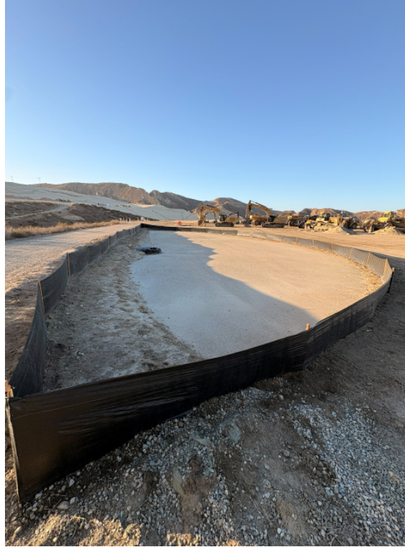
Photo 3. Repaired Silt Fence Surrounding South Culvert in Canyon B
