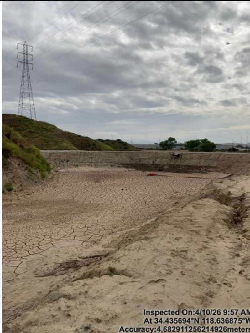
Photo 13 Sub basin 3 installed upgradient of the East Basin
