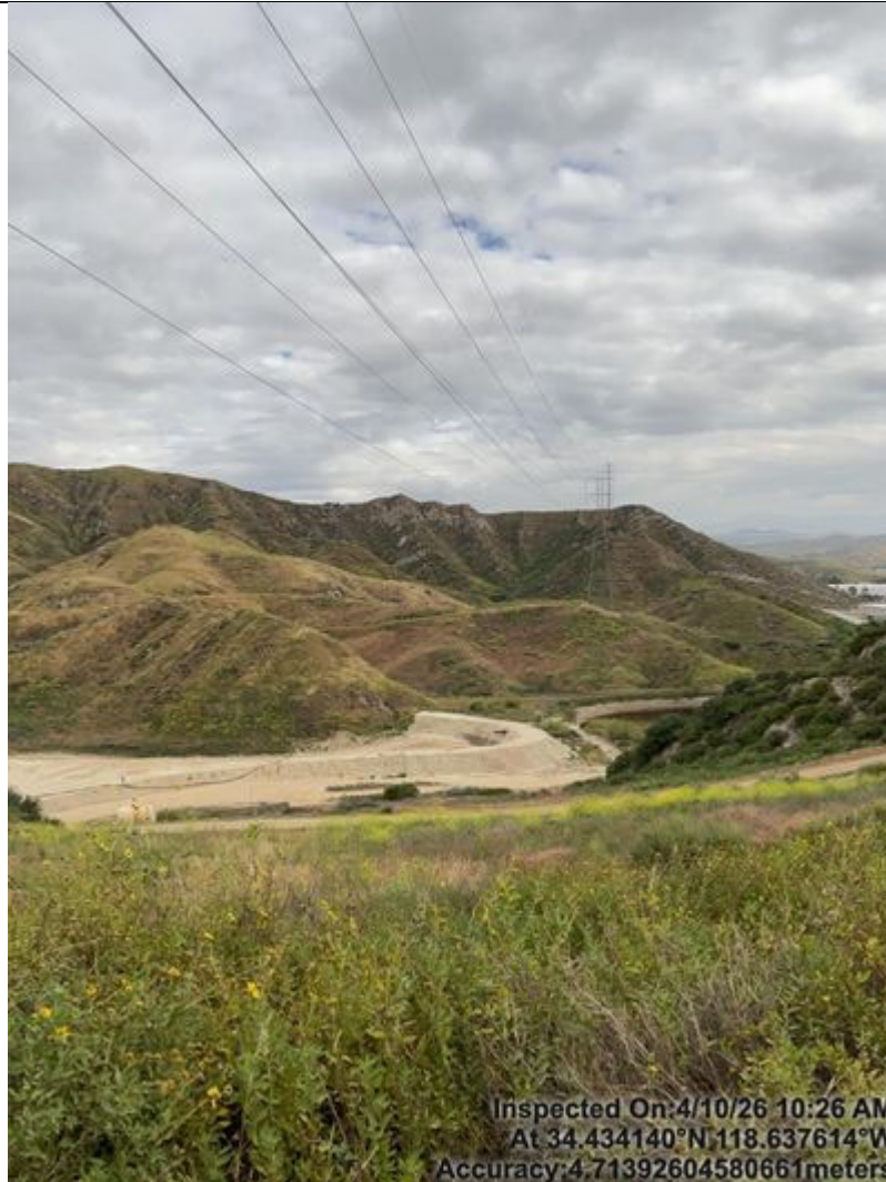
Photo 43 View from culvert outlet to East Basin
