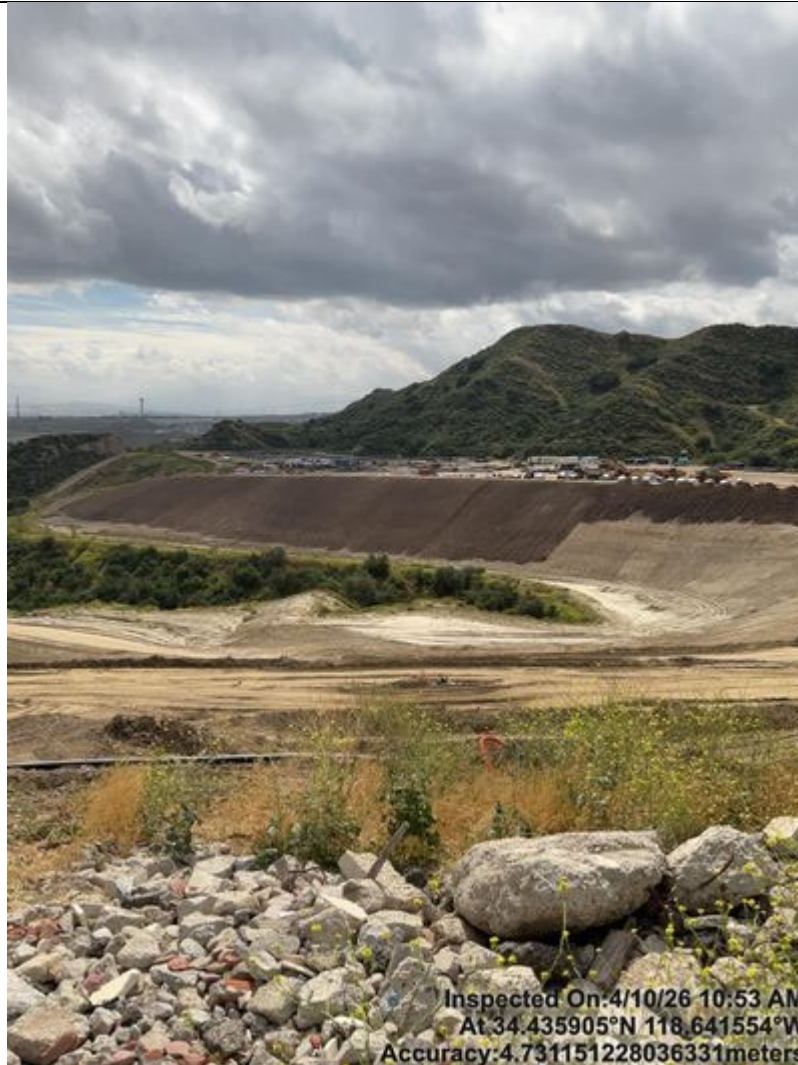
Photo 87 Slope being track walked with fresh media at the northeast end of the Site
