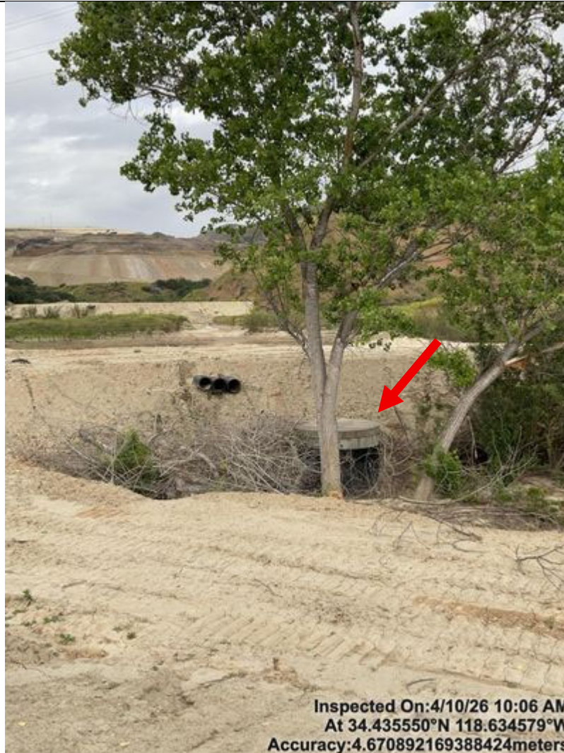
Photo 20 A view of the East Basin. The red arrow points to the covered riser
