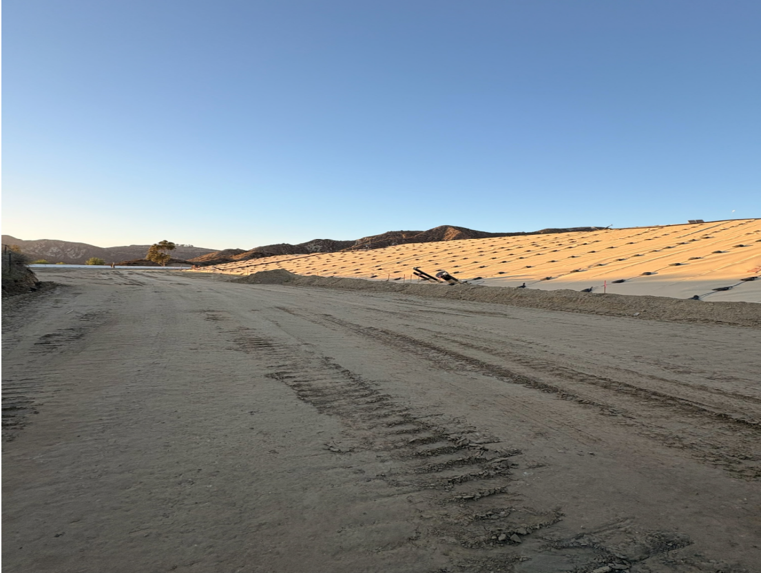
Photo 10. West Toe Area At Location of Former V-Ditch
