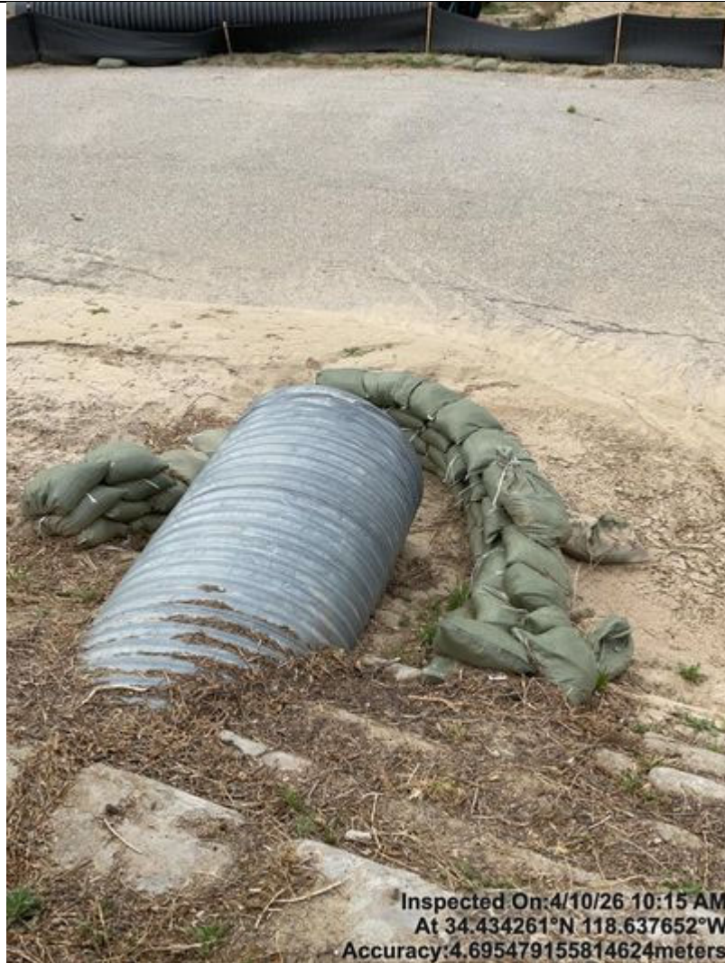
Photo 29 Close-up of the culvert. I observed sediment accumulation around the sandbags
