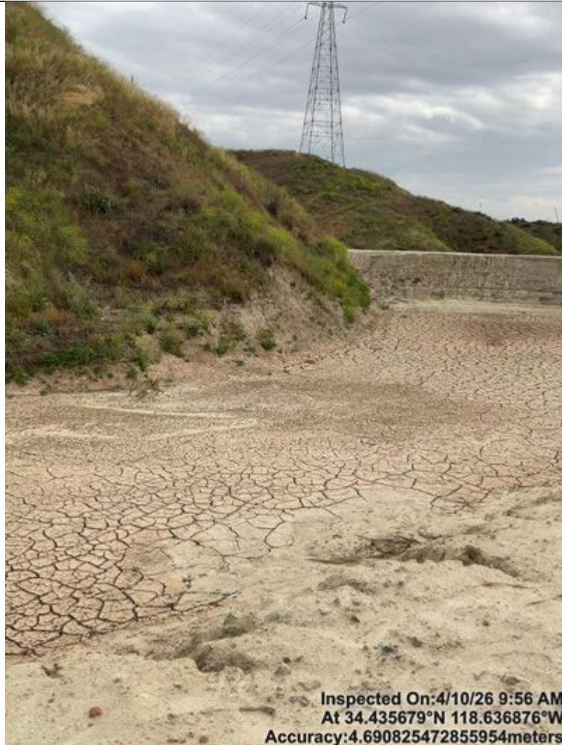
Photo 11 Sub basin 3 installed upgradient of the East Basin
