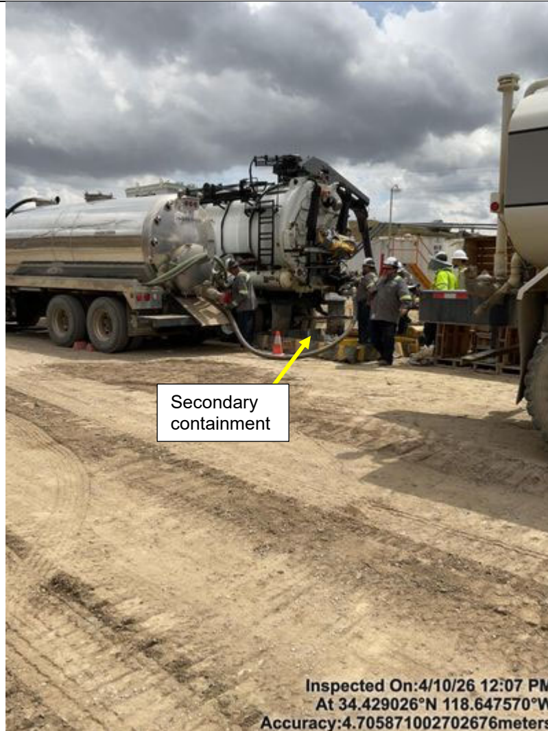
Photo 116 Leachate transfer to vacuum truck
