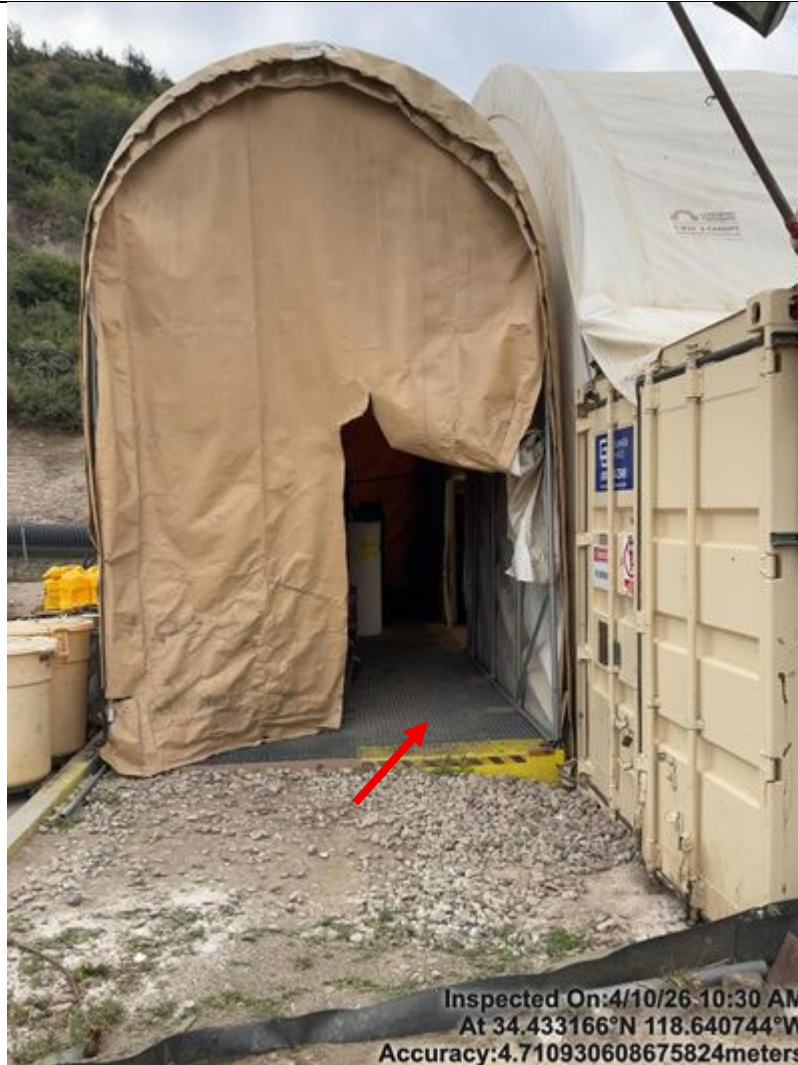
Photo 56 Covered oil storage area with secondary containment grate below (red arrow)
