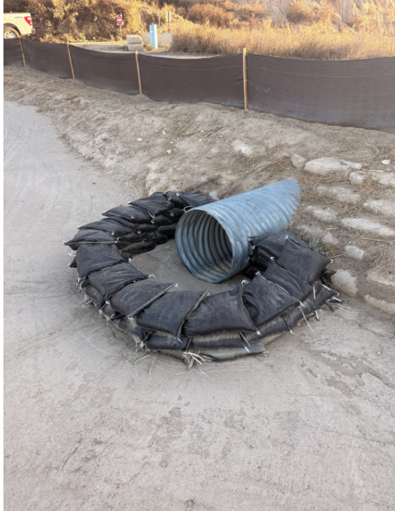
Photo 1. Repaired Sand Bags Surrounding South Culvert in Canyon B
