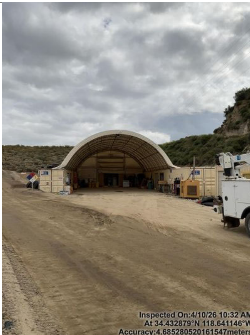
Photo 60 Covered maintenance area
