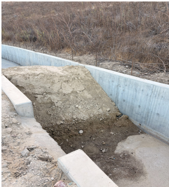
Photo 8. Check Dam in Box Culvert Near West Toe of Landfill
