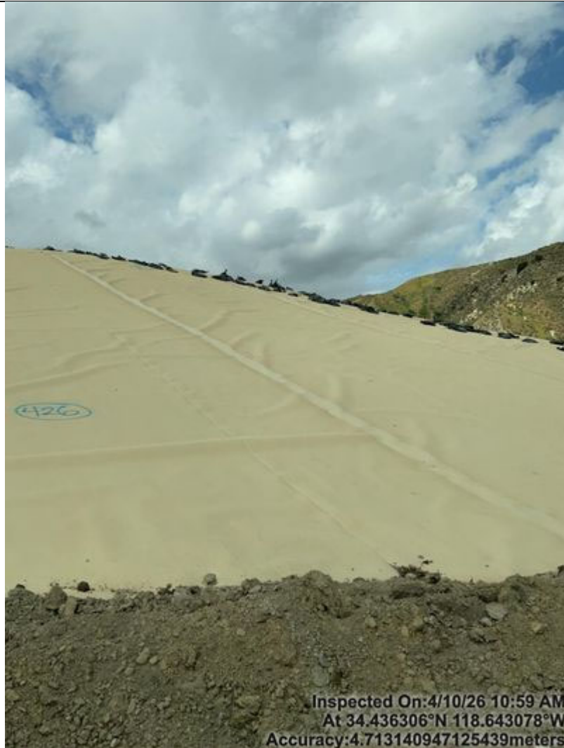
Photo 91 EVOH cover on landfill slopes, required by DTSC
