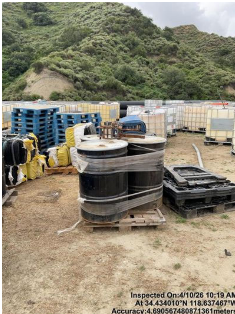
Photo 44 Drum and tote storage outdoors without secondary containment
