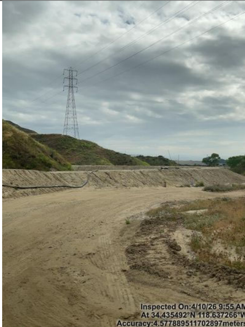
Photo 9 Sub basin 3 installed upgradient of the East Basin
