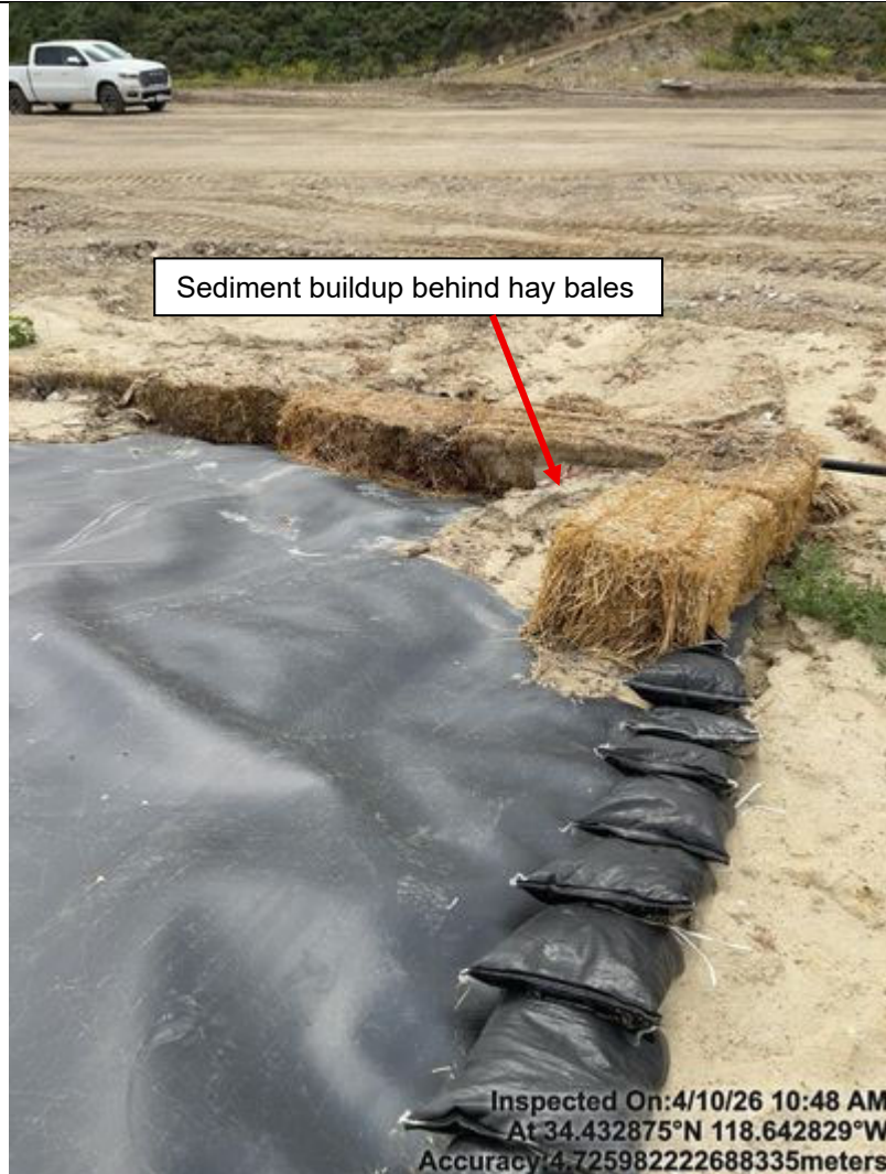
Photo 82 Close-up of erosion control BMP
