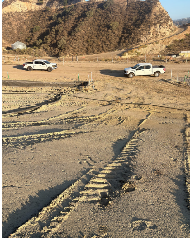
Photo 5. EVOH Preparation Work Near Former Temporary Hay-Bale Erosion Control BMP on East Slope of Main Canyon
