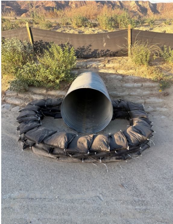
Photo 2. Repaired Sand Bags Surrounding North Culvert in Canyon B
