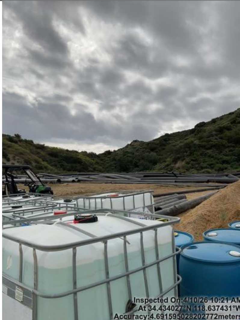
Photo 49 Pipe lay down yard behind totes
