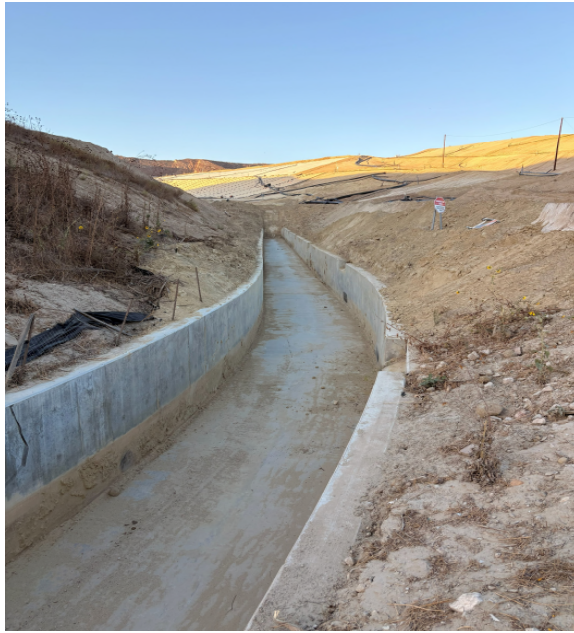
Photo 7. Box Culvert Near West Toe of Landfill
