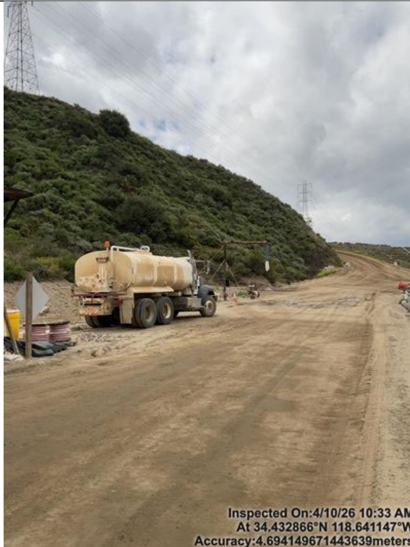
Photo 62 View facing away from the maintenance area
