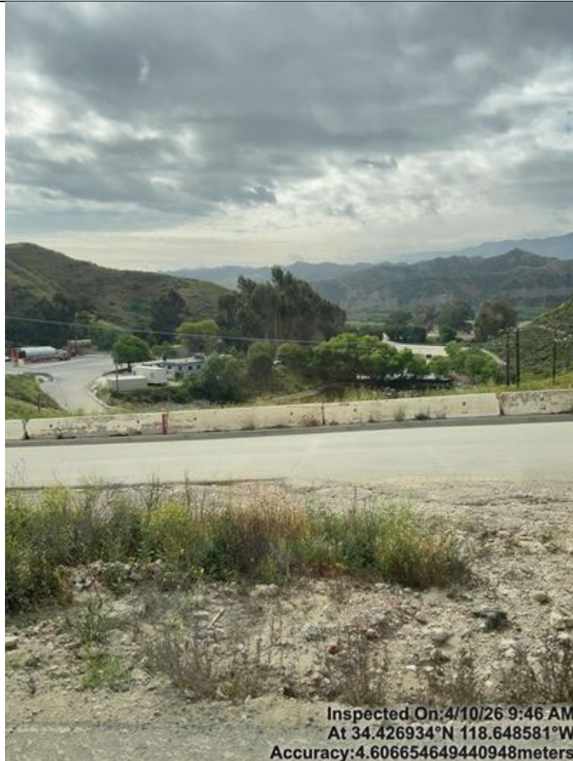
Photo 3 View above the South Basin, facing Henry Mayo Dr
