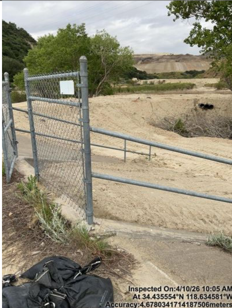
Photo 19 View of the box culvert at the East Basin
