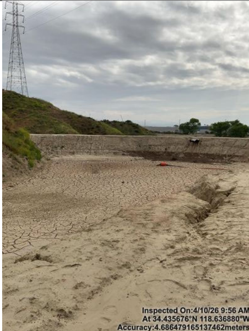
Photo 10 Sub basin 3 installed upgradient of the East Basin
