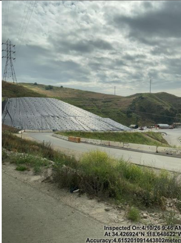
Photo 2 Erosion cover at the south end of CCL
