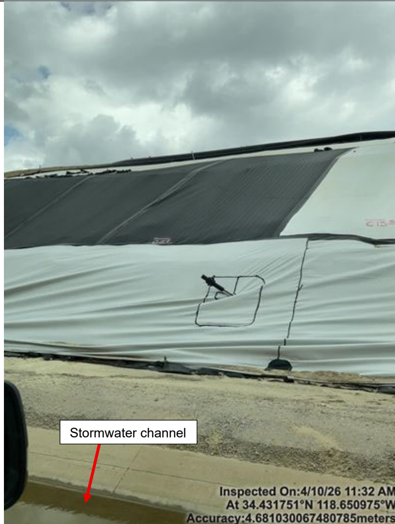
Photo 104 Liner over the west toe slope
