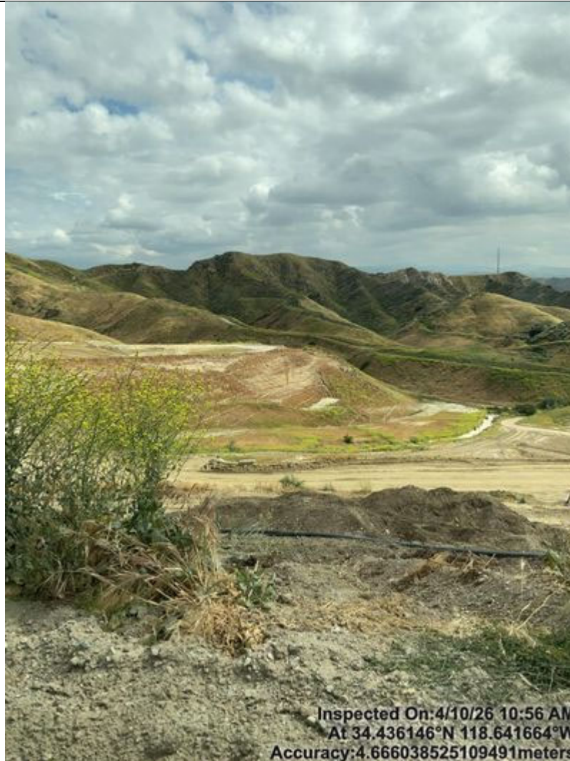
Photo 89 Hydroseeding sloped area. Mr. Breuer stated that this area has CGP coverage
