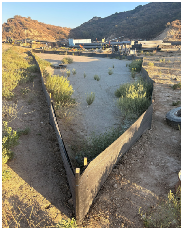
Photo 4. Repaired Silt Fence Surrounding North Culvert in Canyon B
