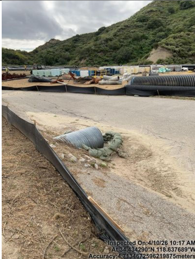
Photo 30 Another view of the culvert and pipe lay down yard
