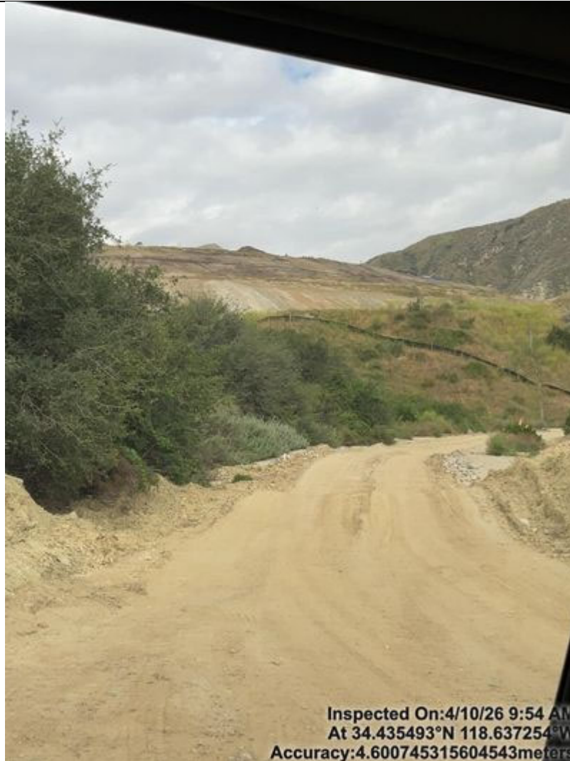
Photo 8 Road approaching sub basin 3, installed upgradient of the East Basin
