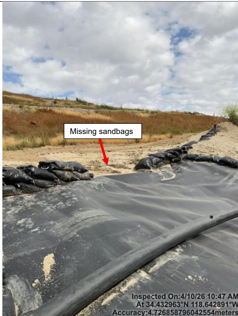
Photo 80 Close-up of erosion control BMP
