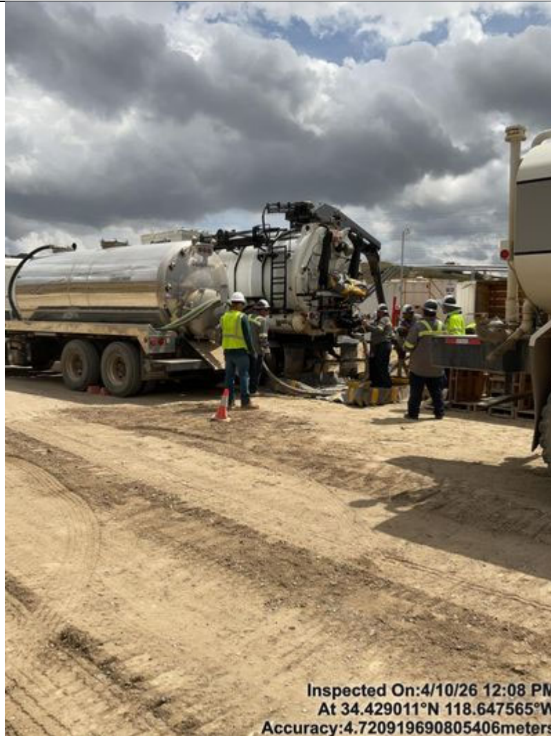
Photo 117 Leachate transfer to vacuum truck
