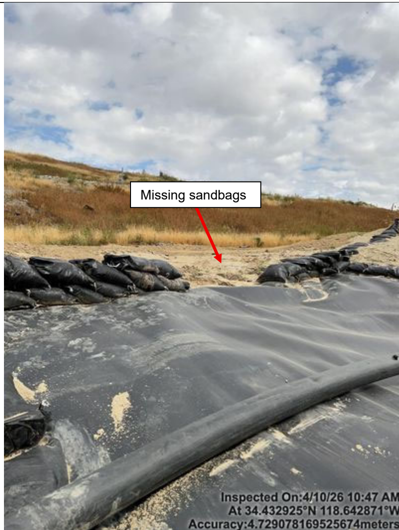
Photo 79 Close-up of erosion control BMP
