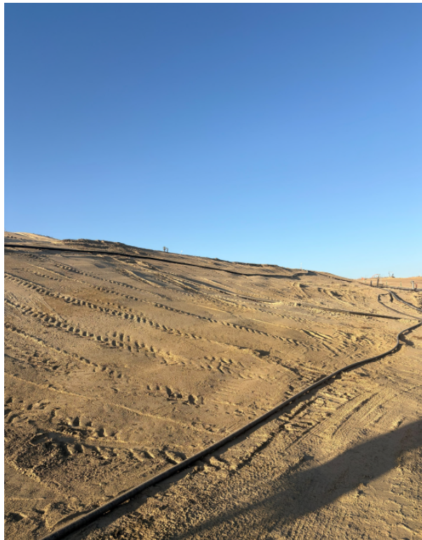
Photo 6. EVOH Preparation Work Near Former Temporary Hay-Bale Erosion Control BMP on East Slope of Main Canyon
