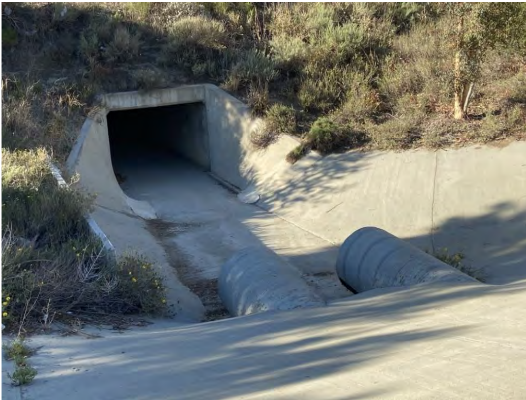
Photograph: Existing Sedimentation Basin Outflow Structures, April 8, 2021.
