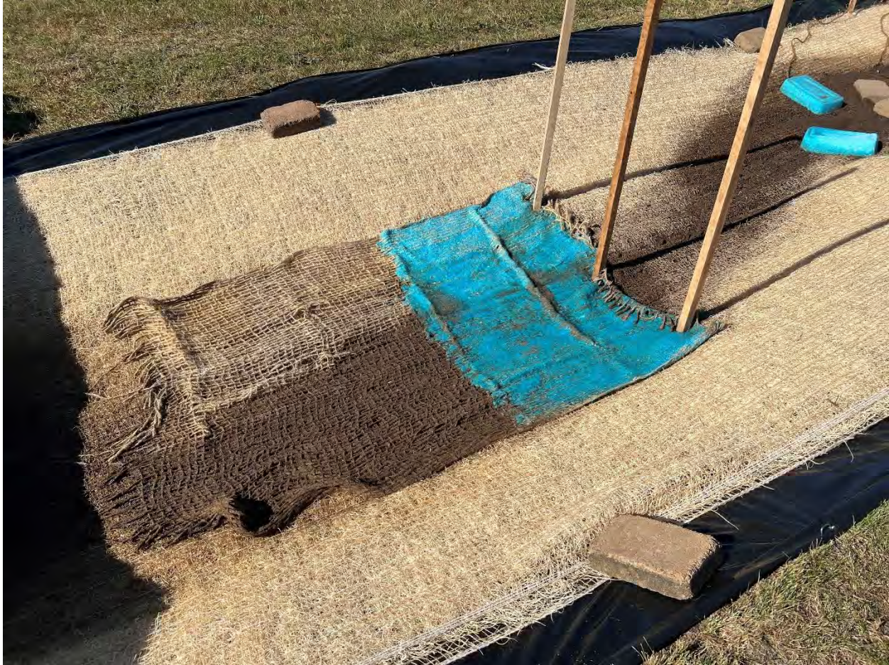
Figure 15 b, c, d. Open Channel Passive Treatment Design examples. Check structures, matting type (as long as rough and fibrous), and rock fill may be changed with other BMPS that promote mixing, flocculation, and particle capture.
