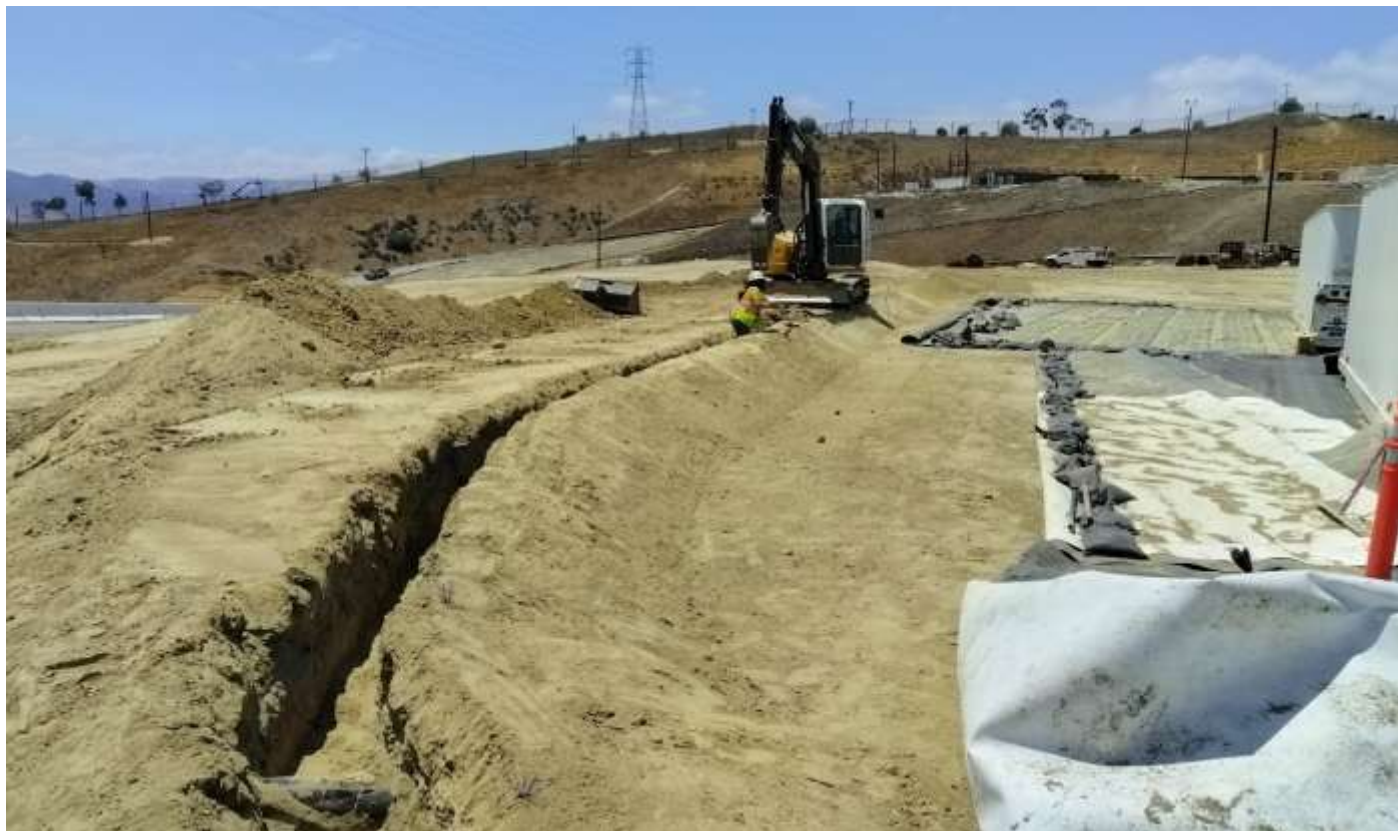
Picture 1: Anchor trench construction (Pad #1).
