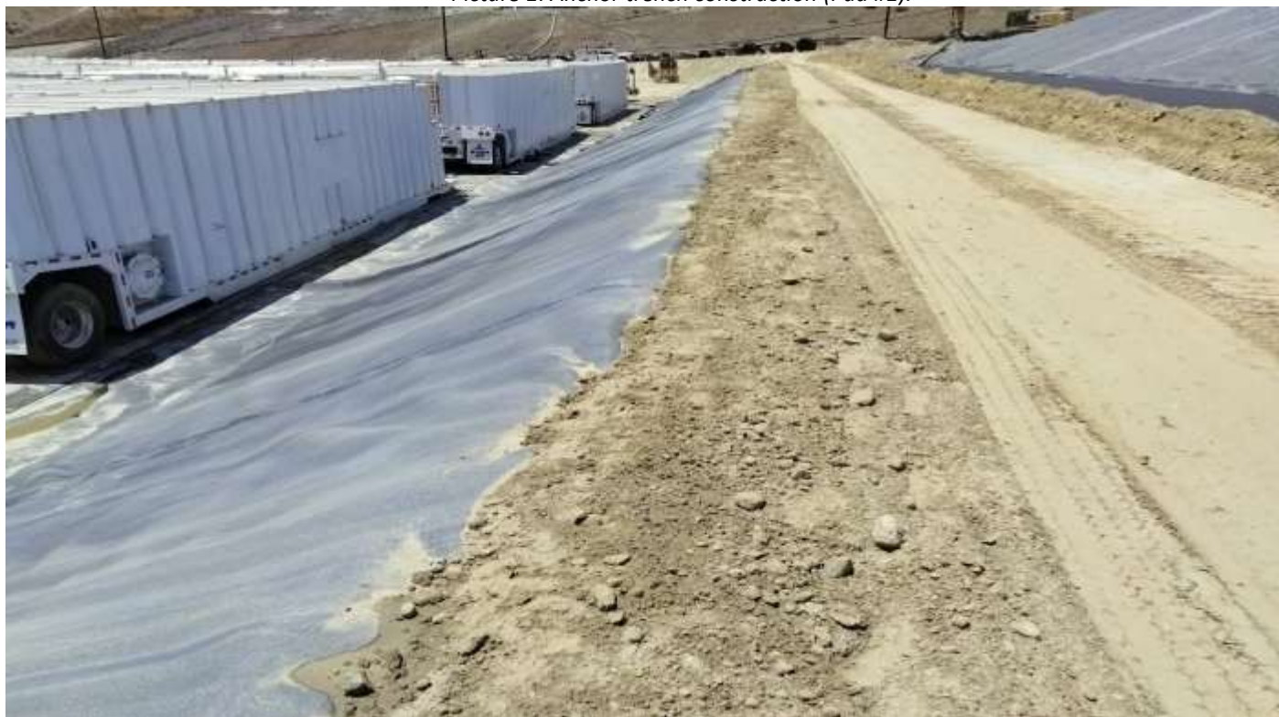
Picture 2: Pad 1 East Slope Backfill
