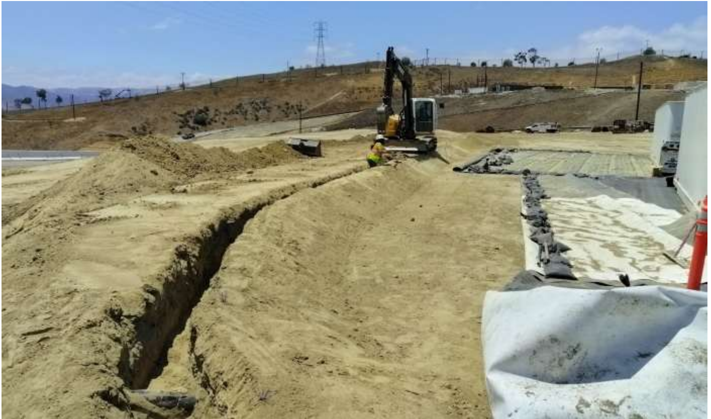
Picture 1: Anchor trench construction (Pad #1).
