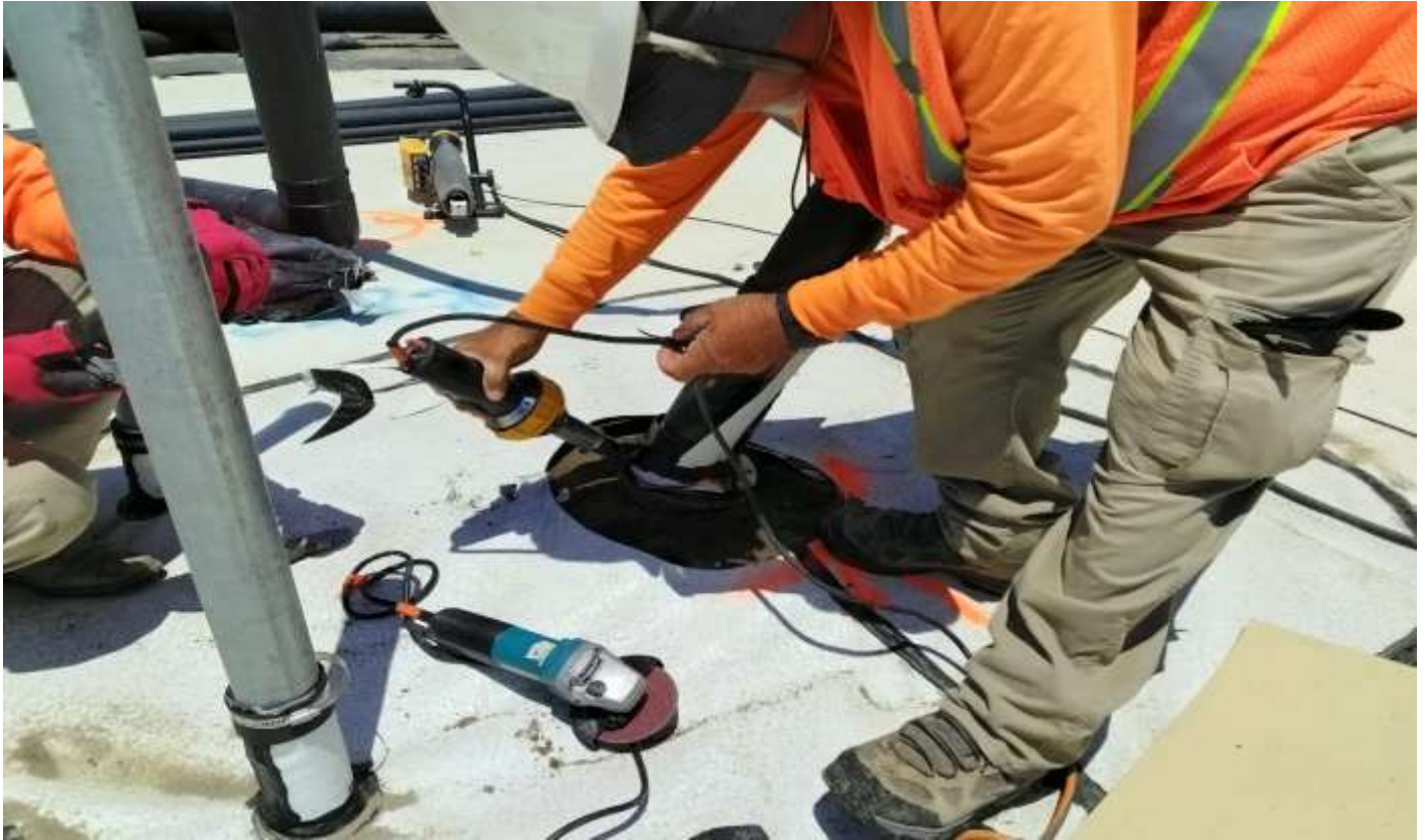
Picture 3: Fabricated Pipe Boots (Top deck)
