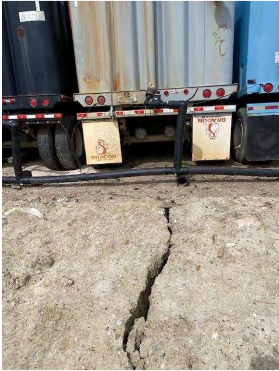
Figure 4. Photograph of tension crack in Grid #148 near leachate tanks on top of CCL dated February 27, 2025 15 .
